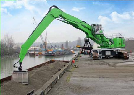
BARGE LOADING FACILITIES
